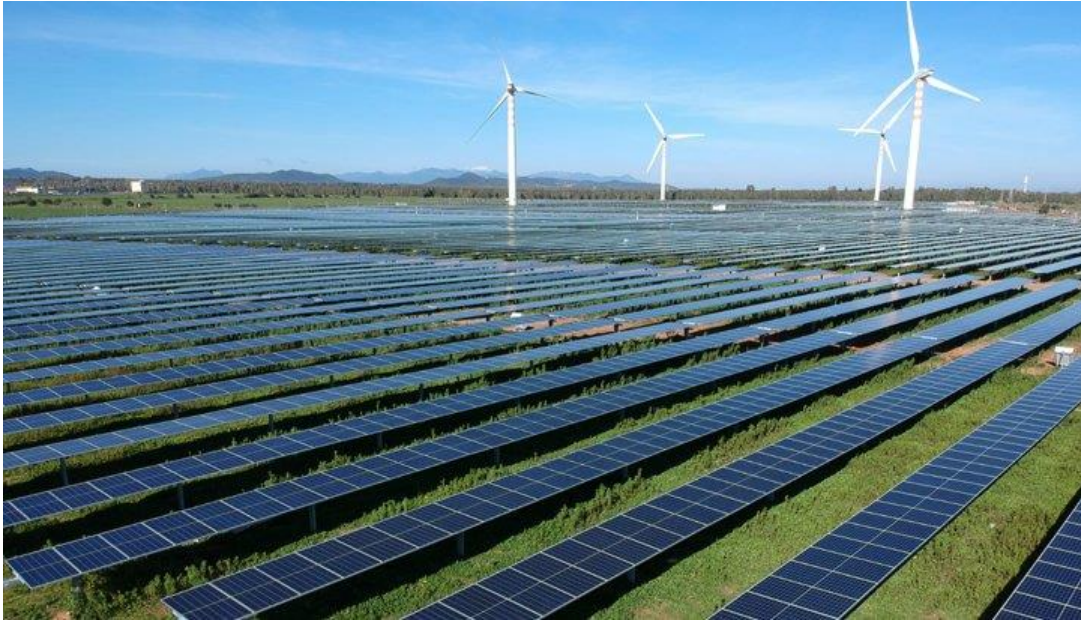
Plate 2: Single Axis Tracker Arrays
